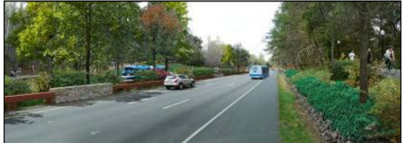
Rural highways can incorporate livability and sustainability principles, such as the multi-use trail, priority bus transit, context-sensitive guardrails, and landscaping shown on the rural highway above.
