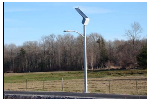
The new pedestrian and bicycle path along Haxton Way, a two-lane rural road in the Lummi Nation near Bellingham, WA provides a safe, attractive alternative to walking along the road. The path is separated from the roadway, using wooden bridges to cross wetlands (above left) and solar lighting (above right).
